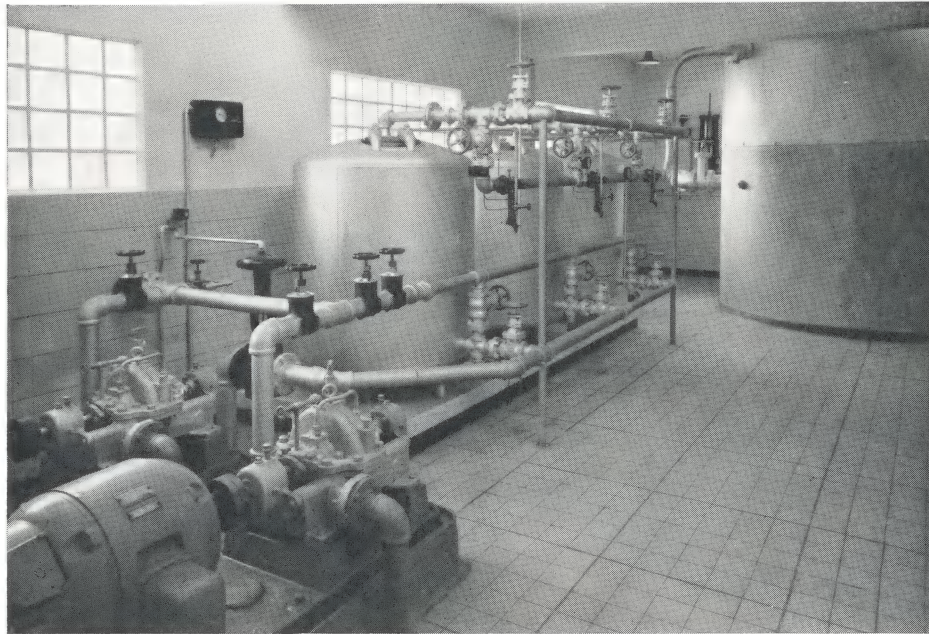
INTERIEUR WATERZUIVERING-STATION HATO MET ACCELATOR EN KOOLFILTERS INTERIOR DI STATION PA FILTRA AWA NA HATO CU ACETELATOR I KOOLFILTER INTERIOR PURIFY-STATION AT HATO WITH ACETELATOR AND CARBONFILTERS
